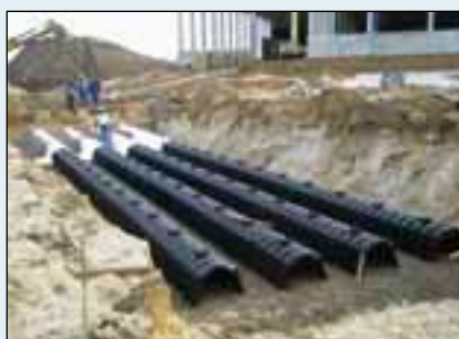
Logistic center, Raben (PL)
